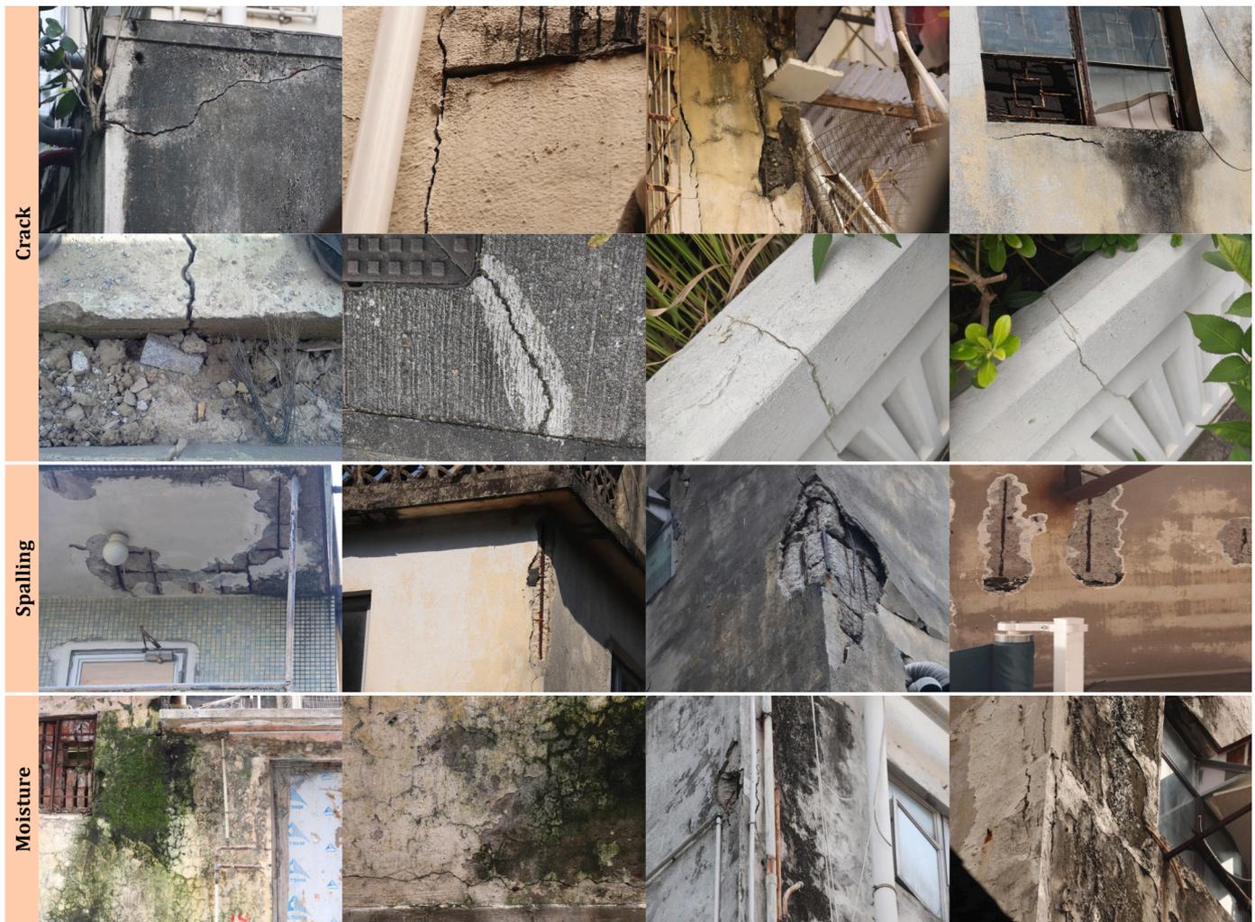
Fig. 2. Sample images from the CUBIT-Det dataset. The first row of images are crack defects on building surfaces and the second row includes crack defects on pavements (first and second column) and bridges (third and fourth column). The third row is about spalling, and the fourth row is about moisture.
