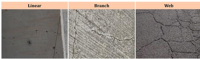
**Fig. 11.** Samples of three different crack labels. “Linear” refers to a single crack; “Branch” is like a branch on a tree but forms a circle; “Web” refers to forming multiple rings and gathering together.
