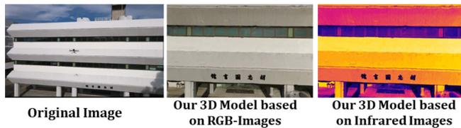
Fig. 3. CUHK United College Wu Chung Library final 3-D reconstruction results based on RGB images and the final infrared 3-D reconstruction results based on infrared images.
